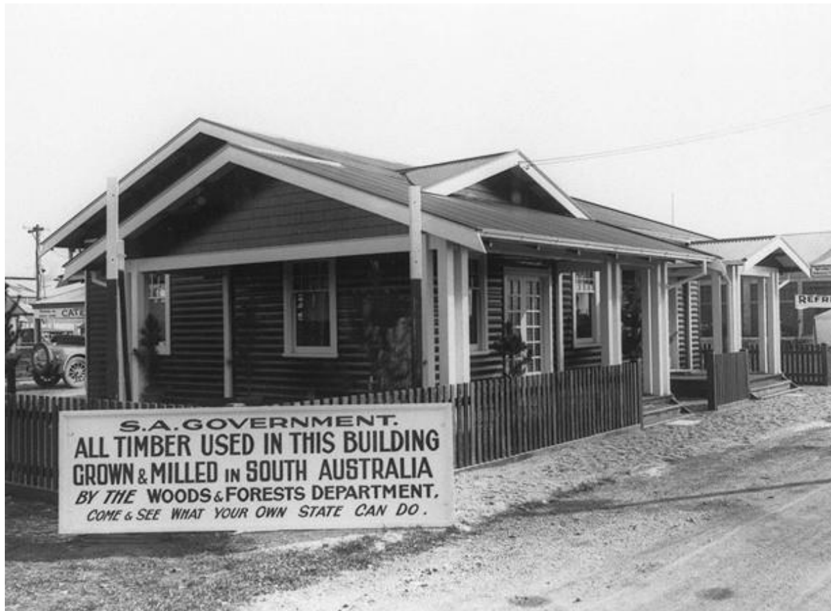
Figure 28: Radiata pine house at the Royal Adelaide Show (1929). The Woods and Forests Department built this full sized house as a demonstration to overcome the resistance to utilisation of radiata pine in housing construction. Source: PIRSA Forestry.
